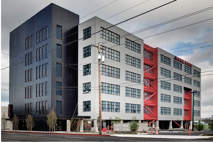
New York Building in Portland
