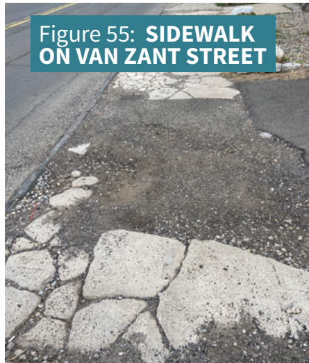
Deteriorating sidewalk conditions on Van Zant Street. Photo taken 3/12/2020.
