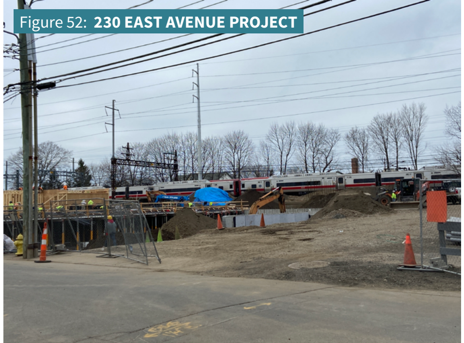
A train passes behind the transit-oriented mixed use development underway at 230 East Avenue. Photo taken 3/12/2020.
