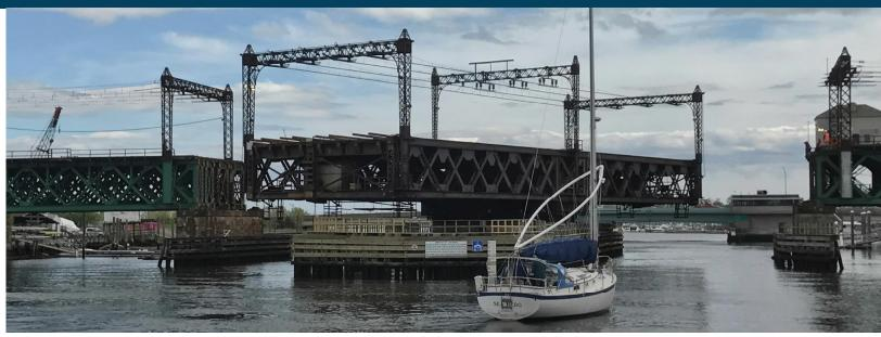
The Norwalk River Railroad (Walk) Bridge was built in 1896 and has outlived its intended service life. It carries four railroad tracks and approximately 175 trains with 125,000 passengers daily. The Walk Bridge has been subject to continued operational failures, is vulnerable to damage from harsh weather conditions, and requires replacement.
